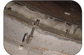
Thorburn's gas turbine expansion joint before turbine washing showing packed thermal insulation
