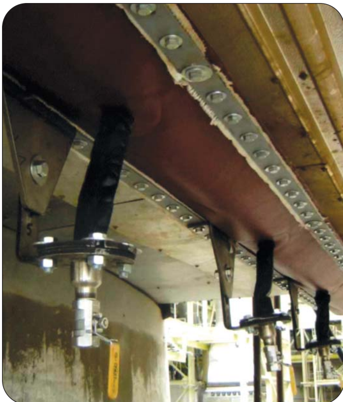
Thorburn's M12 GSM with integral drains on the bottom of a rectangular Flexi-Duct™ expansion joint complete with flex hoses and ball valves at an Egyptian power plant
