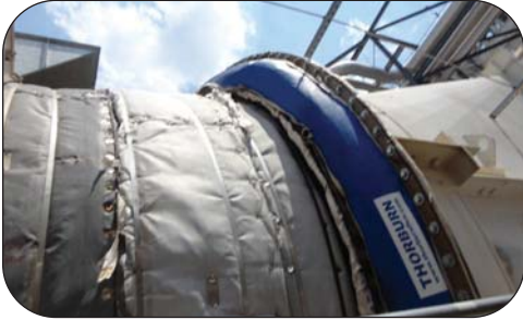
Thorburn installed a Flexi-Duct™ GTEJ-CC gas turbine exhaust expansion joint in Missouri USA
