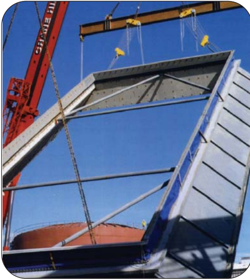
Thorburn's outlet expansion joint being installed at an HRSG in Huntstown, Ireland
