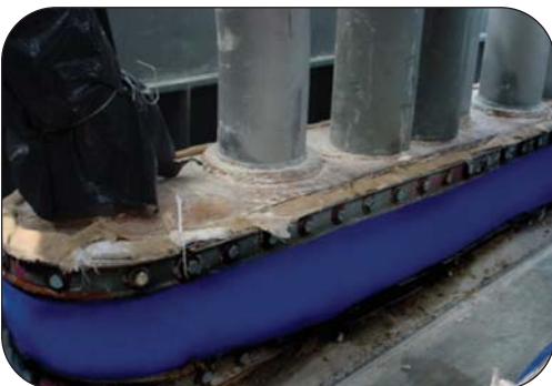
Six non-insulated steam pipes grouped into one Thorburn Flexi-Duct™ penetration seal expansion joint at a Florida power plant
