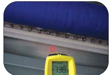
Thorburn's Site team measuring the temperature of an expansion joint's mating structure in an HRSG in Kansas, USA
