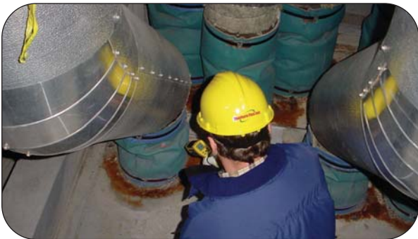
Thorburn's technician recording temperature of a penetration seal at an HRSG in Oregon, USA
