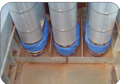
A series of fully insulated dual steam pipes into one Thorburn Flexi-Duct™ penetration seal expansion joint in a Mexican power plant
