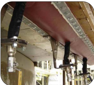
Flexi-Duct™ with M12 GSM and drainage system at a power plant in Alexandria, Egypt
