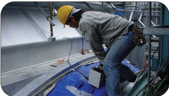
Thorburn Malaysian site team providing training on the proper procedures of splicing a KLF GSM at Malaysian gas fired power plant
