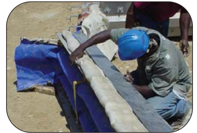
Thorburn's site team inspecting a section of a Flexi-Duct™ expansion joint before final assembly at a gas fired power plant in Australia
