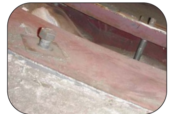
Thorburn's gas turbine expansion joint after turbine washing showing compacted insulation creating a cavity
